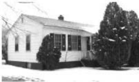
1144 HOUSTON AVE. FOUNDATION OWNED - RENTAL
