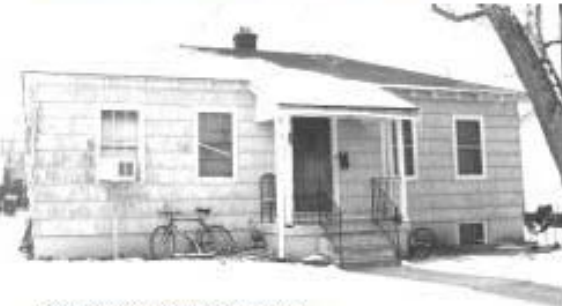
1210 HOUSTON AVE. FOUNDATION OWNED - RENTAL
