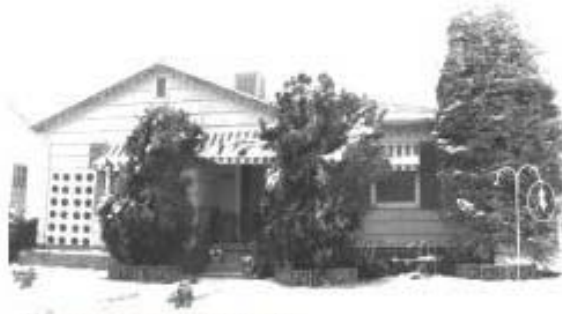
1136 HOUSTON AVE. FOUNDATION OWNED - RENTAL
