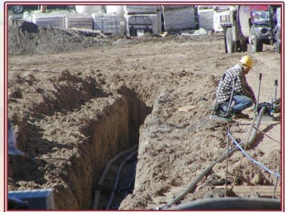
Pipes connecting bore holes
