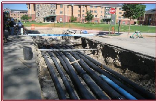
8" dia. Pipes between Central Loop And H.H
